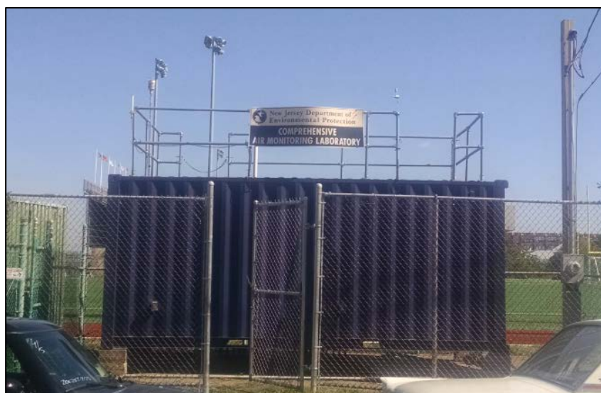
Figure 2-1 Bayonne Air Monitoring Station
